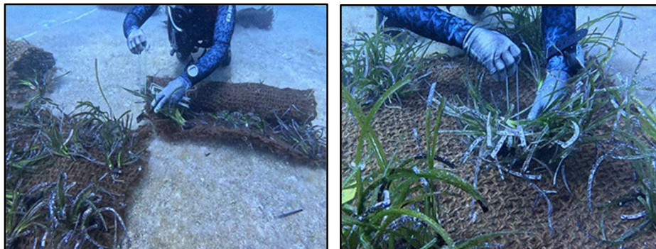
Figure 1.6. View of underwater activities during coconut mats fixation on the substrate.
